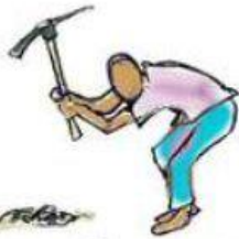
1. DIG TWO HOLES 18IN DEEP AND ABOUT 2FT APART
